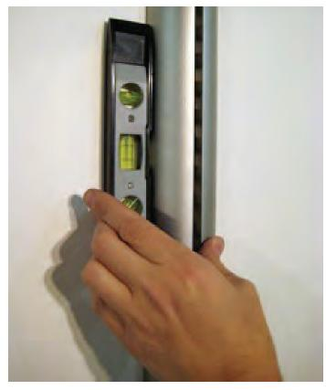
**Tip:** Every once in a while you will run into a stud and your drywall anchor will not screw in all the way. In this case, you can bypass the drywall anchor by taking it out and just directly screwing the upright into the wall with the screw.
